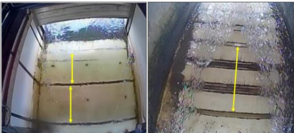
Figure 2 – Overhead view of the Turbine House (left) and Fish Pass (right). The distance between neighbouring electrodes, as indicated by each yellow line, is 45 cm.
